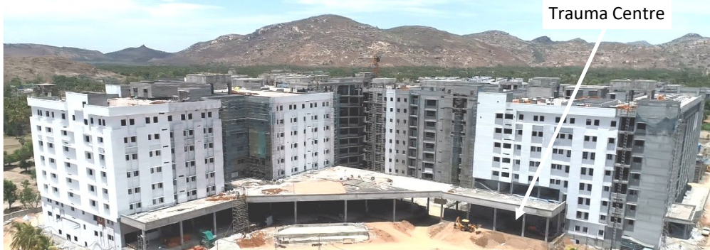
Kannigapuram hospital nearing completion
