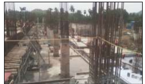
Buildings taking shape at Kannigapuram
