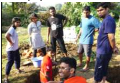
Students dig toilets: Jawadahi camp
